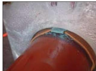
Corrosion to earth shim of CT
